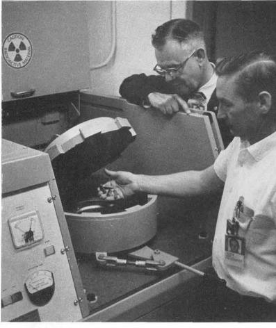
LEAD-LINED TANK, which later will be filled with Kr-85 gas, is part of new leak-detection apparatus. John L. Hutton (7322) and A. R. Elwell (7323) load tank with components to undergo test.
